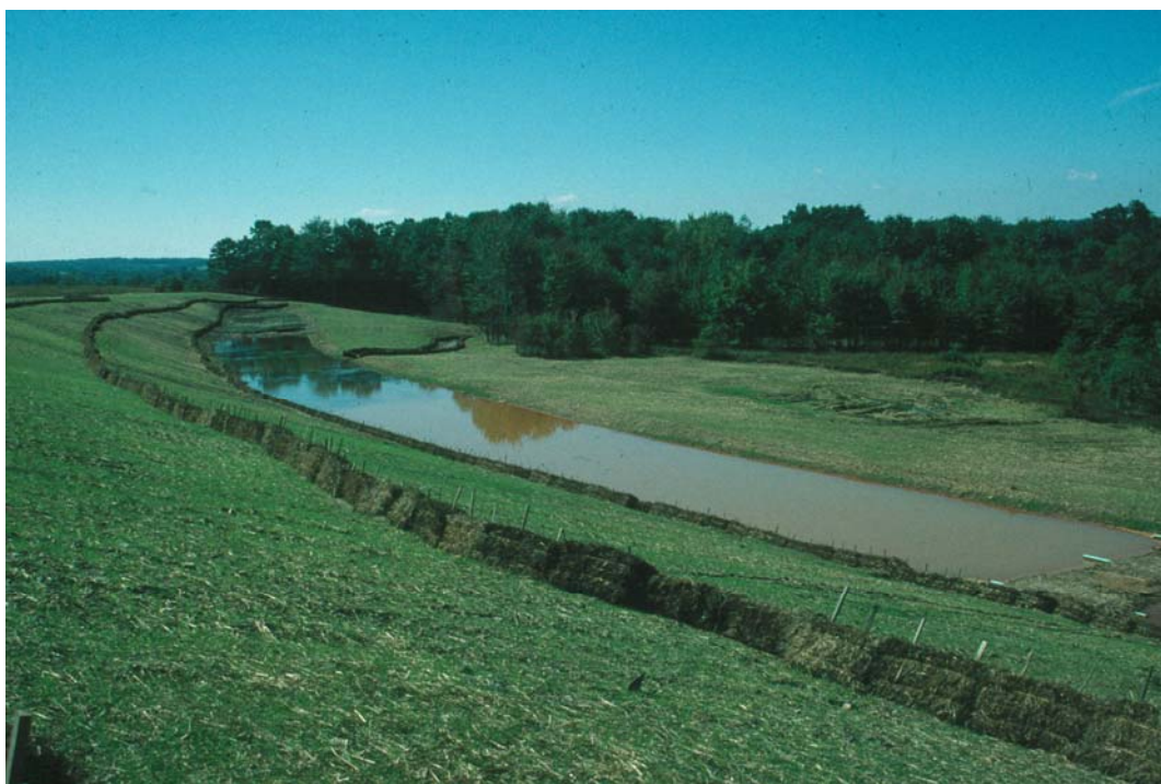
Figure 2. The WV-4b anaerobic wetland systems (AnW). This wetland system removed 3.9 \text{ g/m}^2/\text{day} .
