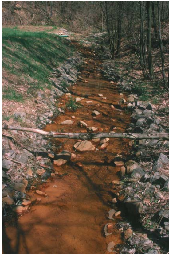
Figure 8. The WV-14 OLC is armored by iron hydroxides, but still has removed an average of 76 g/day/t of acidity. The channel is on a slope of about 15% and receives the drainage from an underground portal. It also receives the runoff from the surrounding hillside, which provides an opportunity for the iron coatings to be flushed during high flow events.
